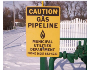
Example of a natural gas pipeline marker.
